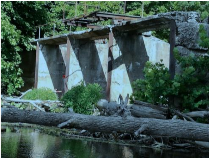
Spillway of the Bingham Mills Dam
