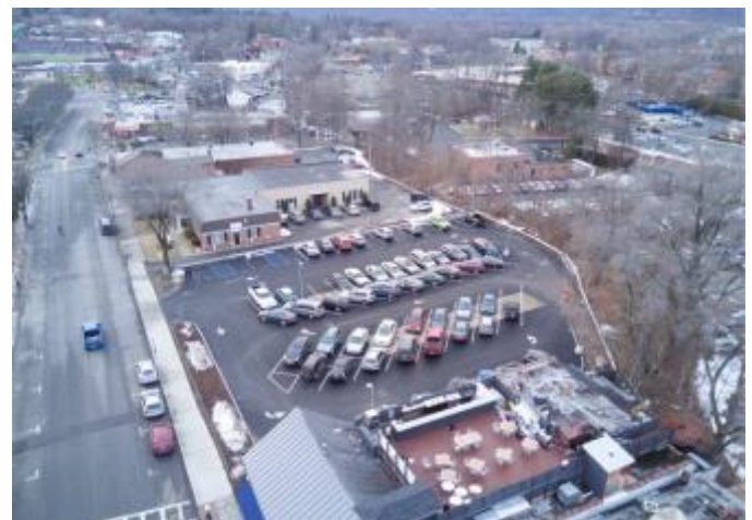
Kingston parking lot and green infrastructure practices (Shawn Willis, Notice Pictures)
