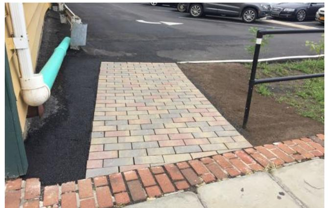
*Figure 4: Series of photos showing the progression of an informal walkway to a formal walkway through Bioretention Area South 1. From top to bottom, photos were taken on 1/1/17, 1/6/17 when gravel was installed, and 7/14/17 when block pavers were installed. This area was originally part of the stormwater practice, and the walkway reduces its designed storage capacity (photos by E. Vail).*
