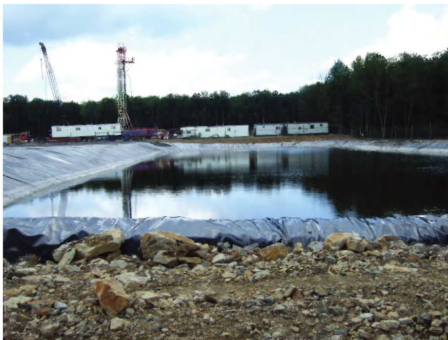
Close-up of Marcellus impoundment, Clearfield County, Pa.
